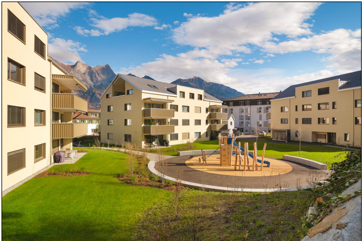
Neubau "Florapark", Bad Ragaz
